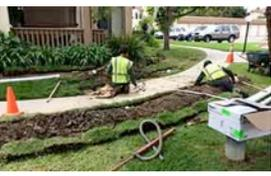
A new rain drainage subsystem has been installed at the northwest corner of Cabana Building. Residence had
