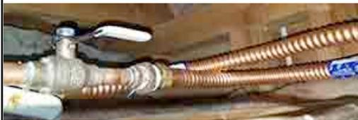
replace. Upgrading with flexible piping with a disconnect, provides easier service.
